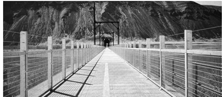
East–West Bridge over the Columbia River at Beverly Washington
