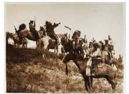
The same photo after repair
