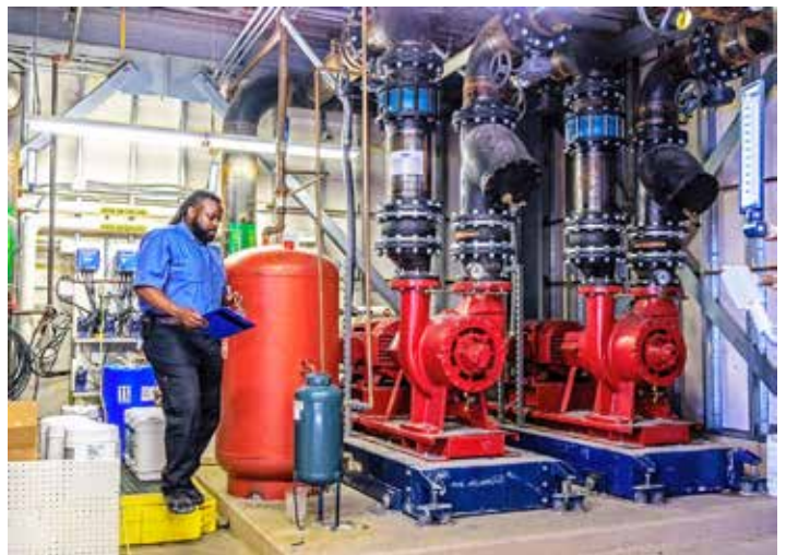
Jamaal Hopkins inspecting the boilers – photo, E. Hill
