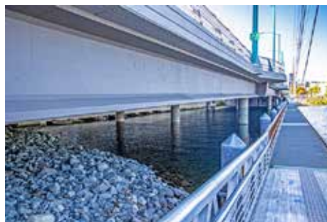
Footbridge at water level – photo by E. Hill
