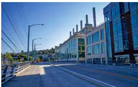
Fairview Ave N Bridge – photo, E. Hill
