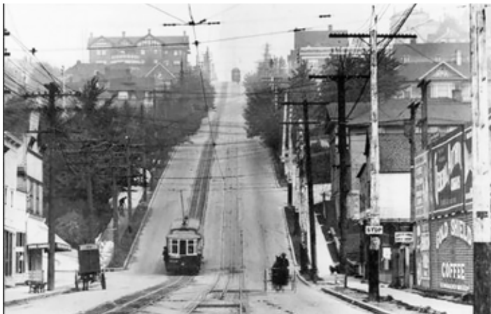
From 1898 until August 10, 1940, streetcars (here seen in 1910) made their way between upper and lower Queen Anne Hill, assisted by a weighting system called a “counterbalance.” Courtesy of Counterbalance Barbershop
